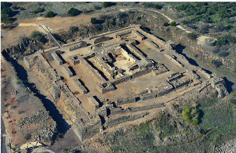
Fig. 4 – Aerial view of Belvoir Castle (Source: https://en.wikipedia.org/wiki/Belvoir_Castle_(Israel) ).
