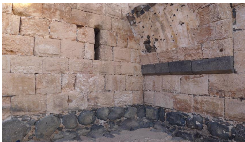
Fig. 6 – Vault inserted in the wall.
