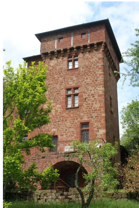
Fig. 2 – Tower of the house of Les Landes in Mouret (Aveyron) (©Y. Mattalia).
