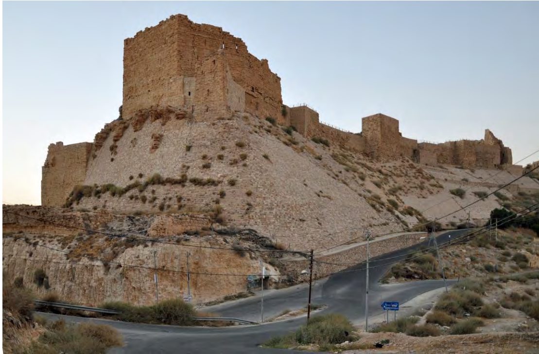
Fig. 1 – Karak Castle: view looking N along the E wall. The Hospitallers’ barbican would have extended from near the tower in the centre of the wall to the now largely demolished NE corner-tower beyond it (© DP 2017).
